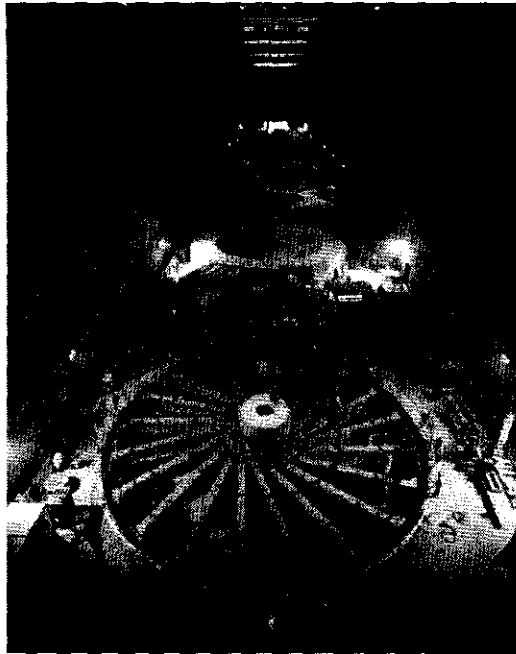
Sanxia inside Powerhouse
