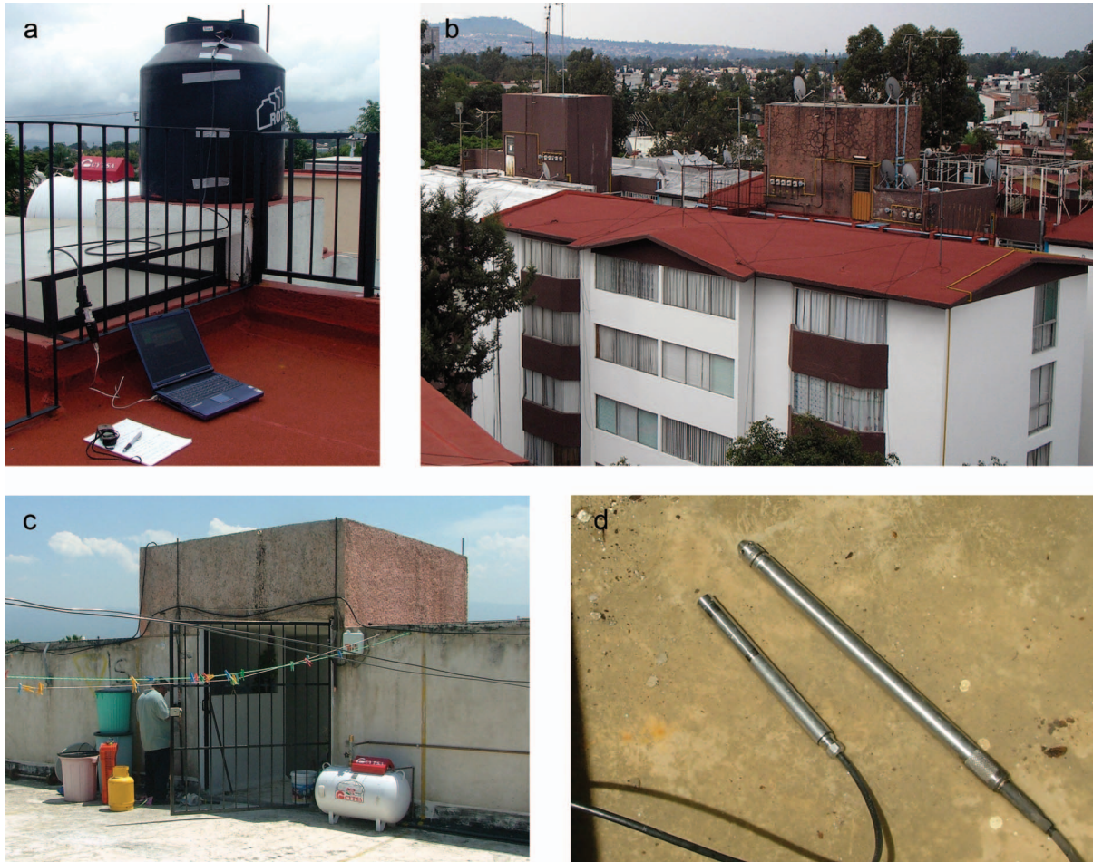
Figure 3. Leak determination in buildings with a roof tank: (a) roof tank on the “Almost empty house” and the “Occupied house,” (b) roof tank on “Building 0”, (c) roof tank on “Building I” and “Building II” and (d) instruments to monitor the water level in the roof tanks.
