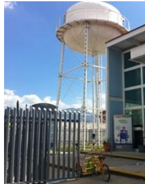
Tanque Carrillo Puerto
